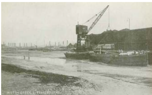
Loading bricks at the dock At Milton Creek
